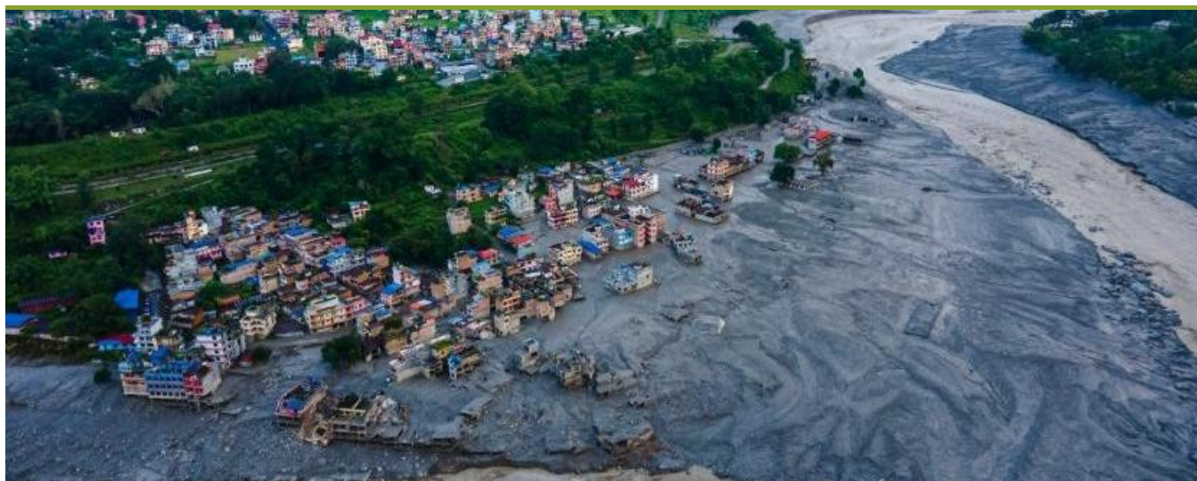
Flood-affected settlement along the Bhotekoshi-Trishuli river corridor following the 26 August 2026 flash flood. Image source: Nexpher News, extracted 20 September 2026
