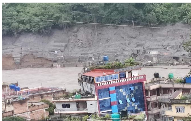
Figure 1. Flood-damaged residential structures and debris along the river corridor.
